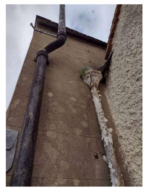
2. The storm water drainage to the rear of the property requires urgent attention, the hopper is blocked and allowing rainwater to cascade down the face of the building.
